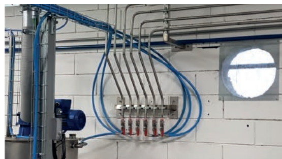
Installed delivery and recirculation line treated with Nitrogen flushing
